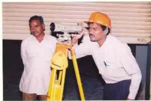
Crane testing in progress
